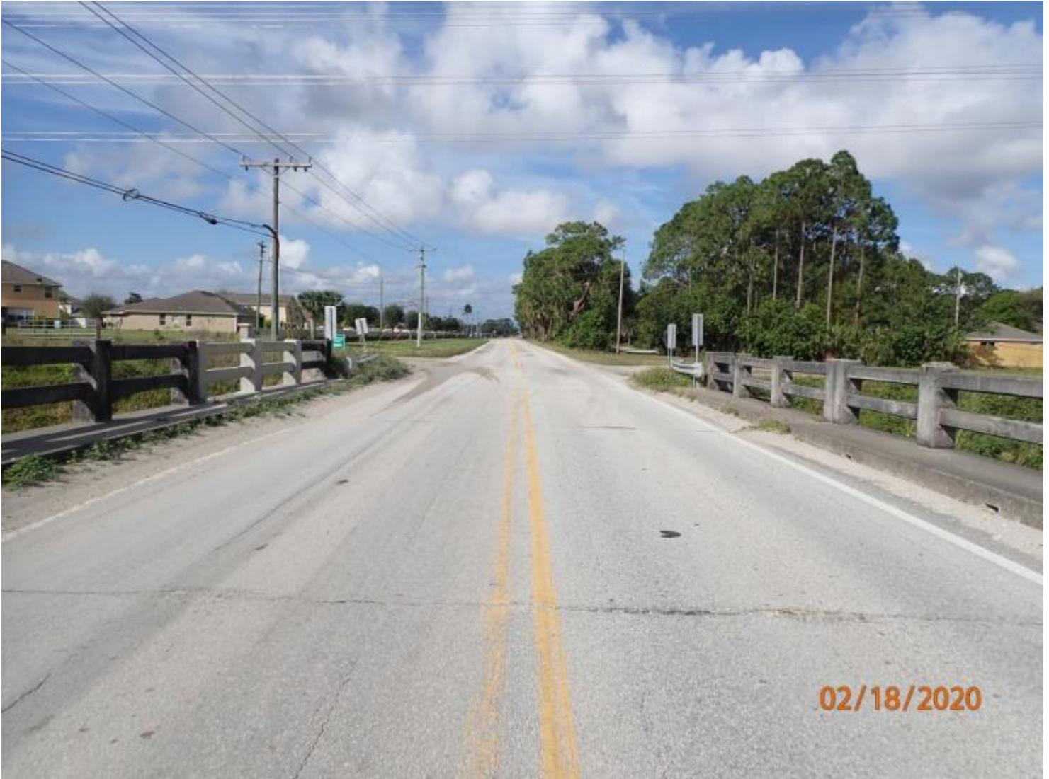
West Approach Looking West
