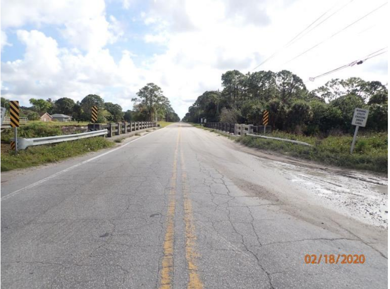
West Approach Looking East
