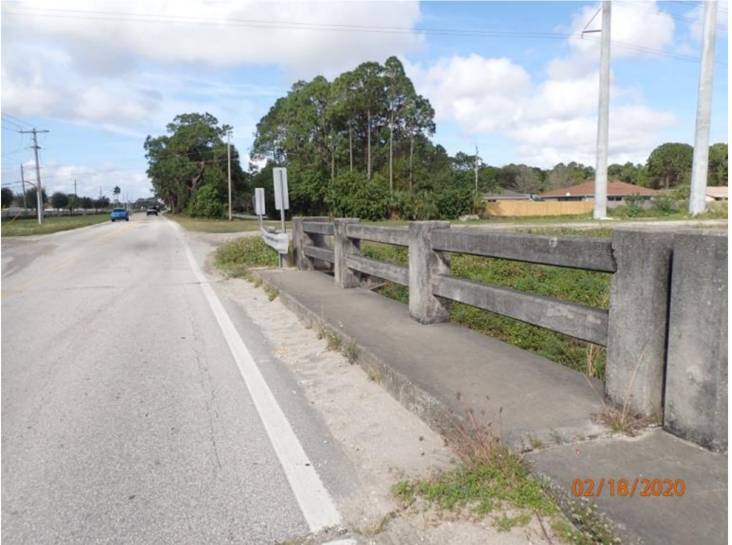
Northwest Off-Going Transition
